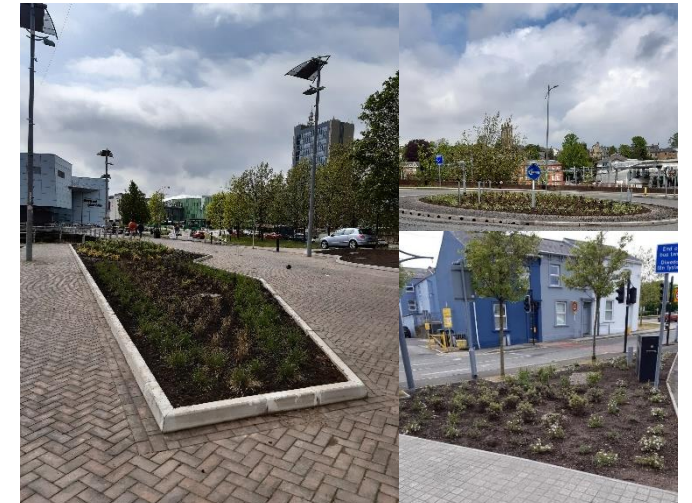
After GI installed
